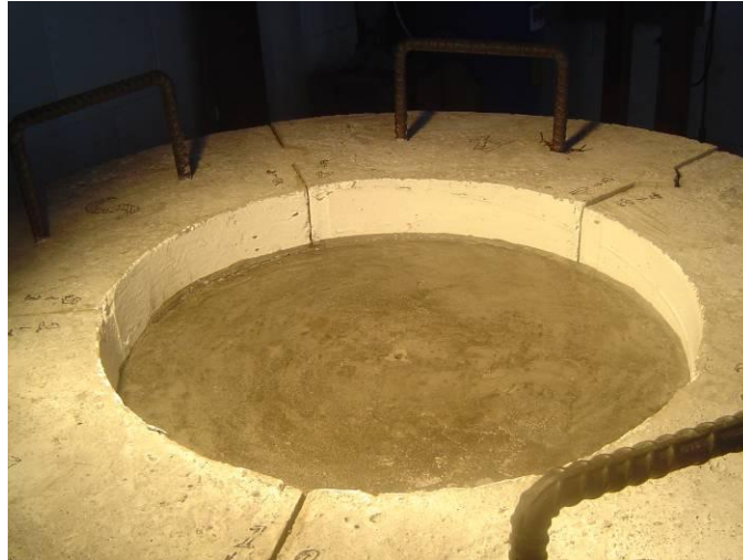
Figure 10.22. Postblast grout sample #7, decoupled 3.6 gram/m detonating cord and confined
